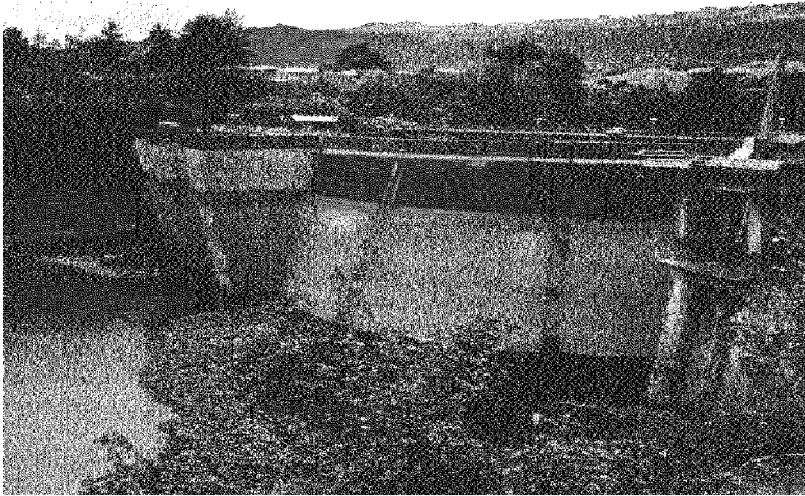
Figure 7-3 View of Cachi dam from upstream.
